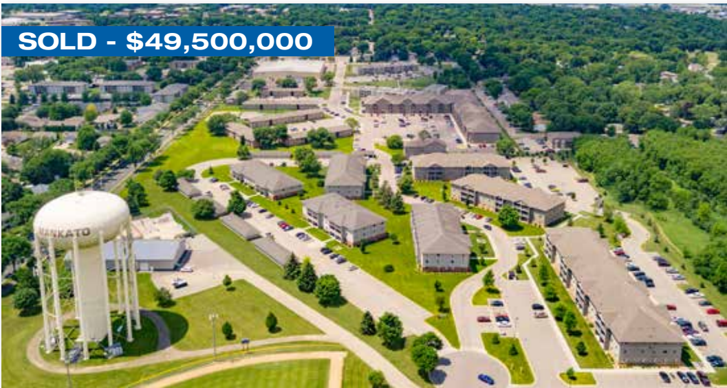
LIVE ACTIVE APARTMENTS 524 UNITS | MANKATO, MN
